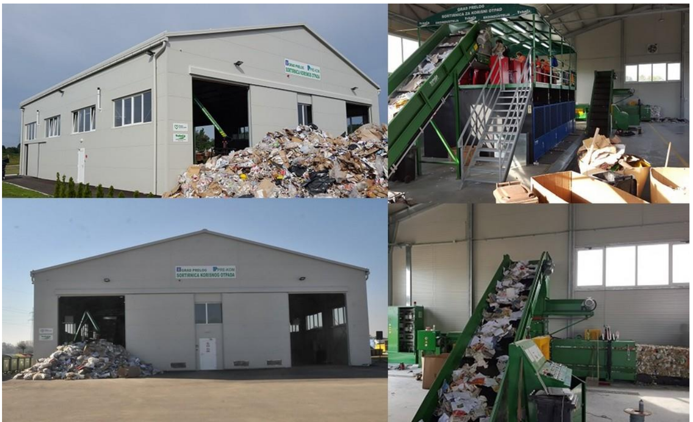
Figure 4 Sorting plant for useful waste in the City of Prelog
