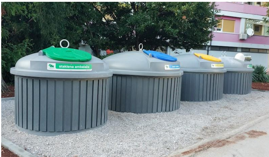
Figure 1 Semi-underground containers for separate collection of waste in the City of Labin
