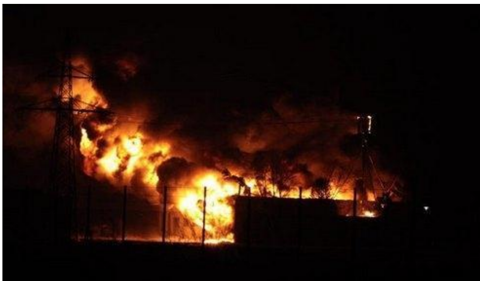
Figure 8 fire broke in the Drava international factory in Osijek (picture: sib.net.hr)
