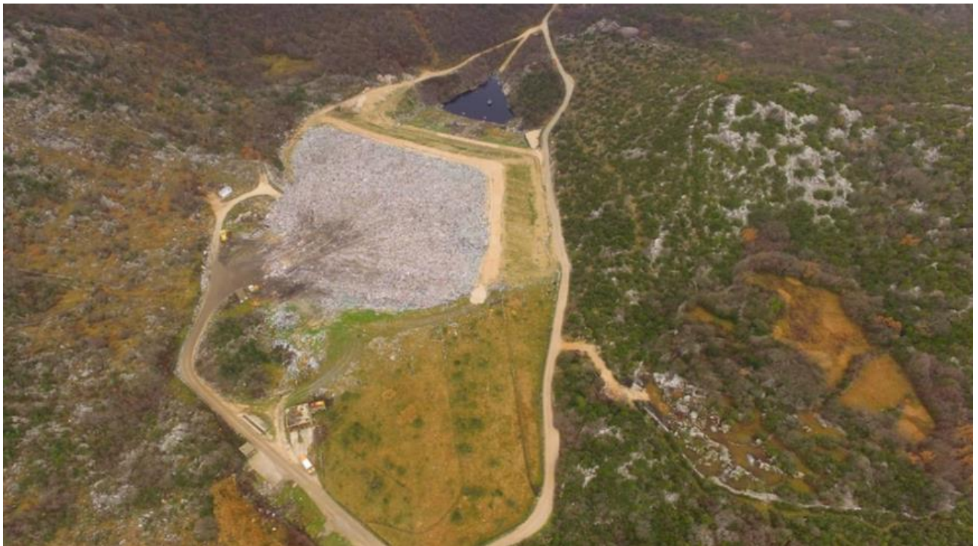
Figure 2. Grabovica landfill (source: City of Dubrovnik)
