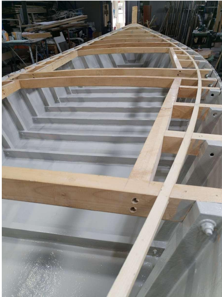
Figure 7 Protection of reconstructed and mounted elements.
