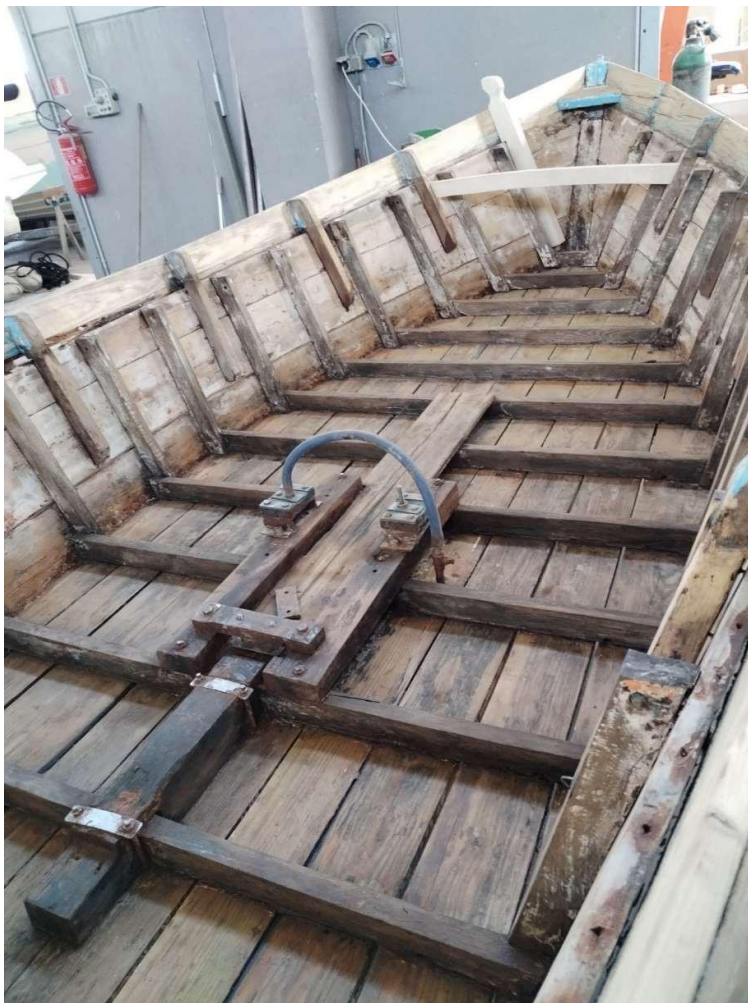
Figure 4 Rotten elements taken off, new elements fitting.
