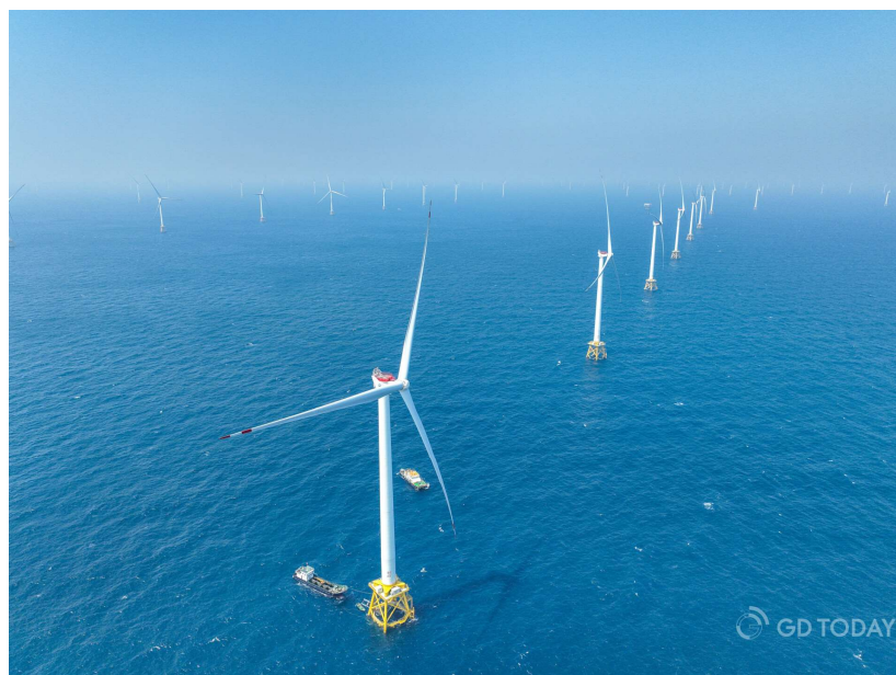
Figure 37 Placement of fish cages and aquaculture nets within the lattice foundation structure of the Mingyu-1 offshore wind farm Source: https://www.newsgd.com/node_e9dced8600/5a39cf85b.shtml
