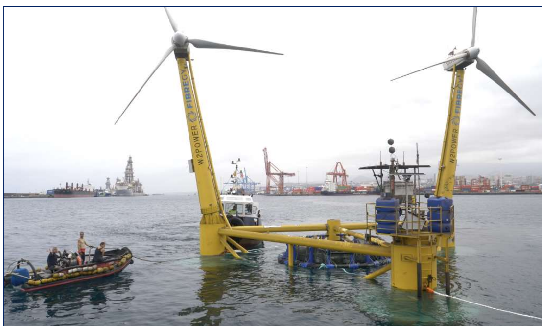
Figure 36 Towing of the multi-use system to its deployment site Source: https://owcltd.com/media/news/aquawind-project-breakthrough-prototype-launch-complete/
