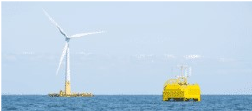
Figure 28 Right: Sealhyfe, pilot project for offshore hydrogen production (Lhyfe) equipped with a Plug electrolyzer, installed on the WAVEGEM platform (GEPS Techno).
