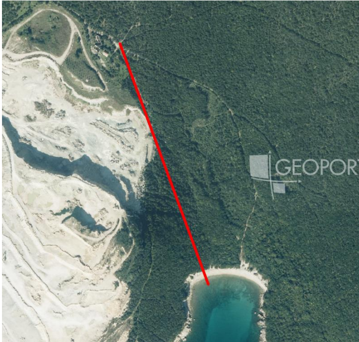
Figure 66 - Position of the longitudinal profile on the orthophoto map for slope stability analyses at Brovinje site.
