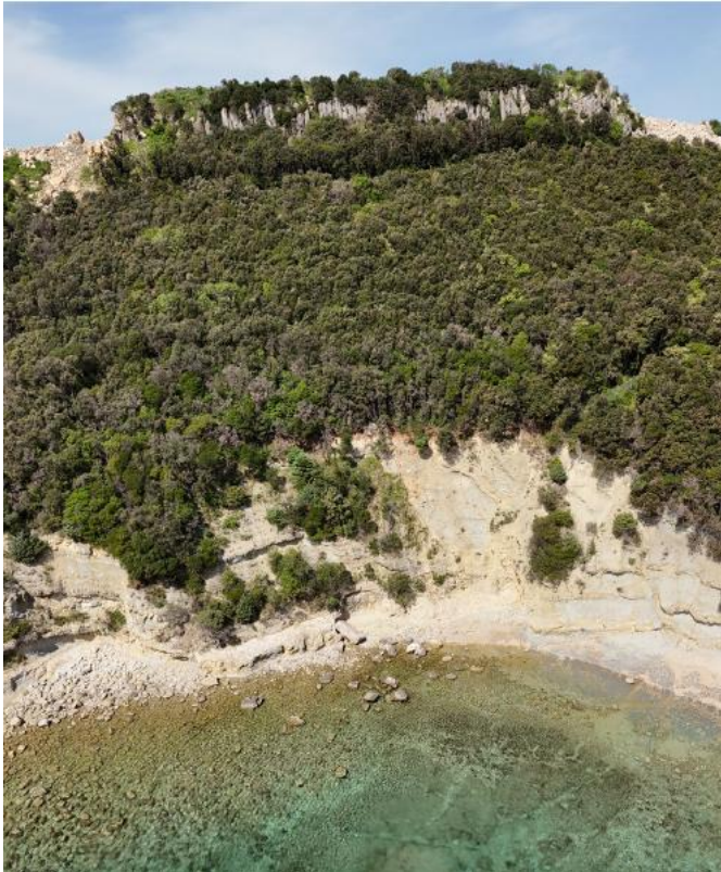
Figure 64 - View of the slope at the Brovinje site.
