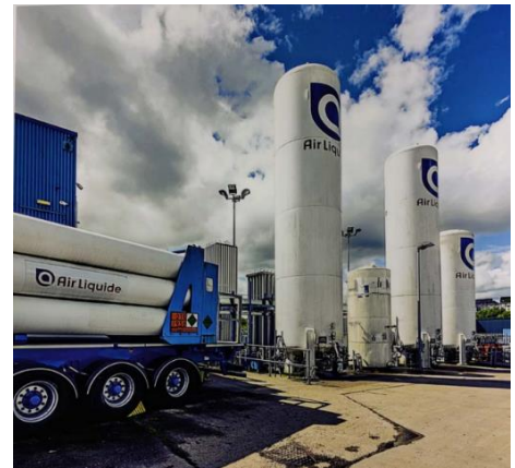
Figure 8-2 Compressed hydrogen tanks
