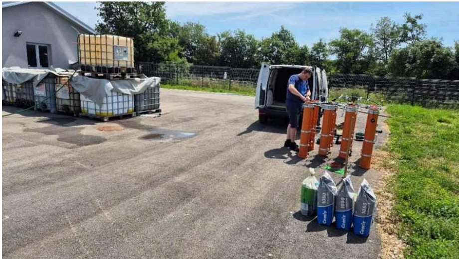
Figure 8. Installation of pilot treatment columns at the Lobarika WWTP site.
