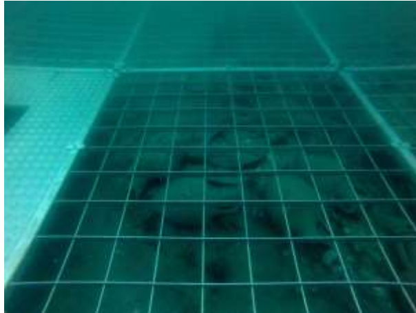
Fig.9 – Positioning of the new grids
