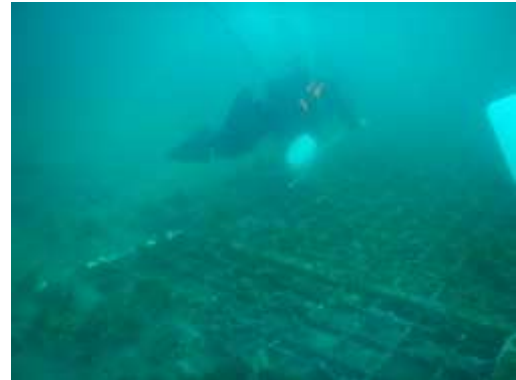
Fig.2 – The removal of the grid
