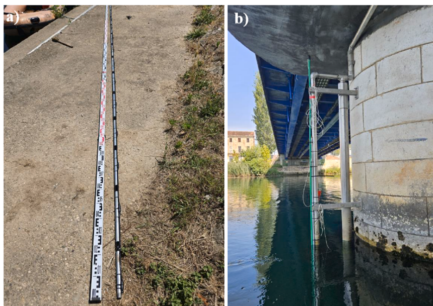
Fig. 3. a) Developed temperature chain consisting of 11 DS18B20 sensors at 40 cm equidistant intervals and b) installed temperature chain at Metković bridge pier in operation.
