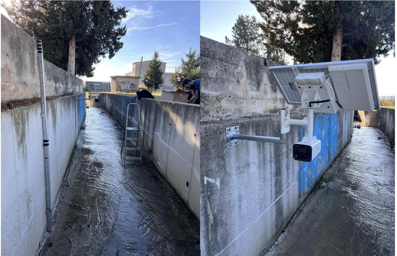
Figure 20. Photographs of mounted camera and installed gauge
